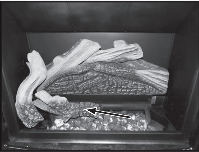
Figure 46: 3rd log placement.
