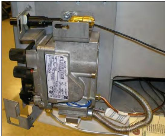
**Step 1:** Disconnect pilot lines and gas supply line from valve on the side of the unit. **NOTE: Care should be taken to ensure that the gas and pilot lines are not damaged during handling. These lines are fragile.**
