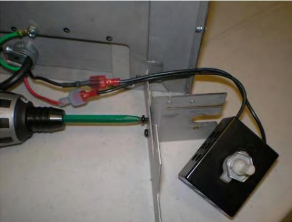
**2** Attach Fan Control Switch Extension Bracket using [2] #6 Combo Screws as shown.
